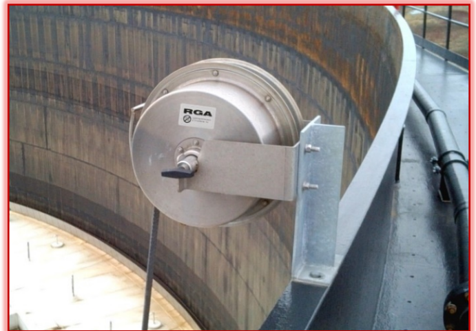
RGA 750 Generation 2 mounted to a vertical standoff bracket* on a floating roof tank.
